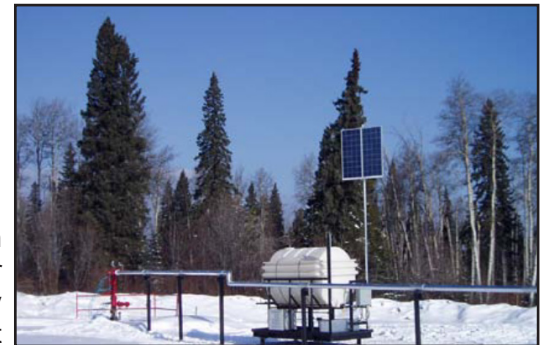
SPEC Injection skid for methanol applications (with stainless pumps)
